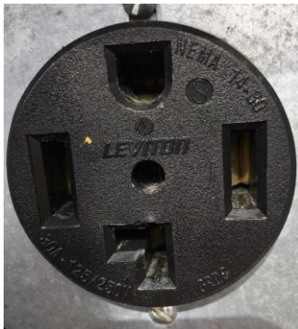
220/30 Amp Outlet. Requires this connection.
