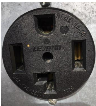
220/30 Amp Outlet. Requires this connection.
