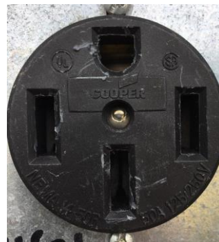
220/50 Amp Outlet. Requires this connection.
