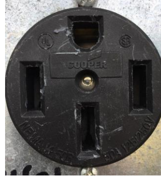
220/50 Amp Outlet. Requires this connection.
