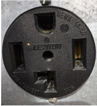
220/30 Amp Outlet. Requires this connection.
