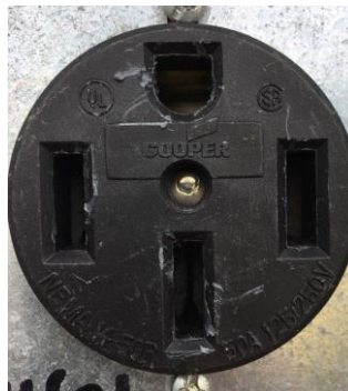
220/50 Amp Outlet. Requires this connection.
