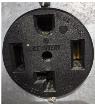
220/30 Amp Outlet. Requires this connection.
